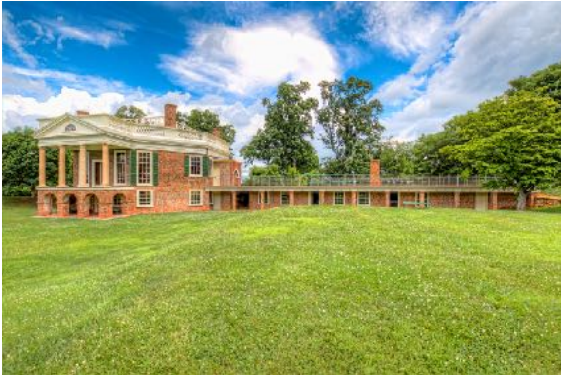
A view from the back of Poplar Forest shows the wing of offices that included a kitchen and smokehouse. Construction on Poplar Forest started in 1806.
