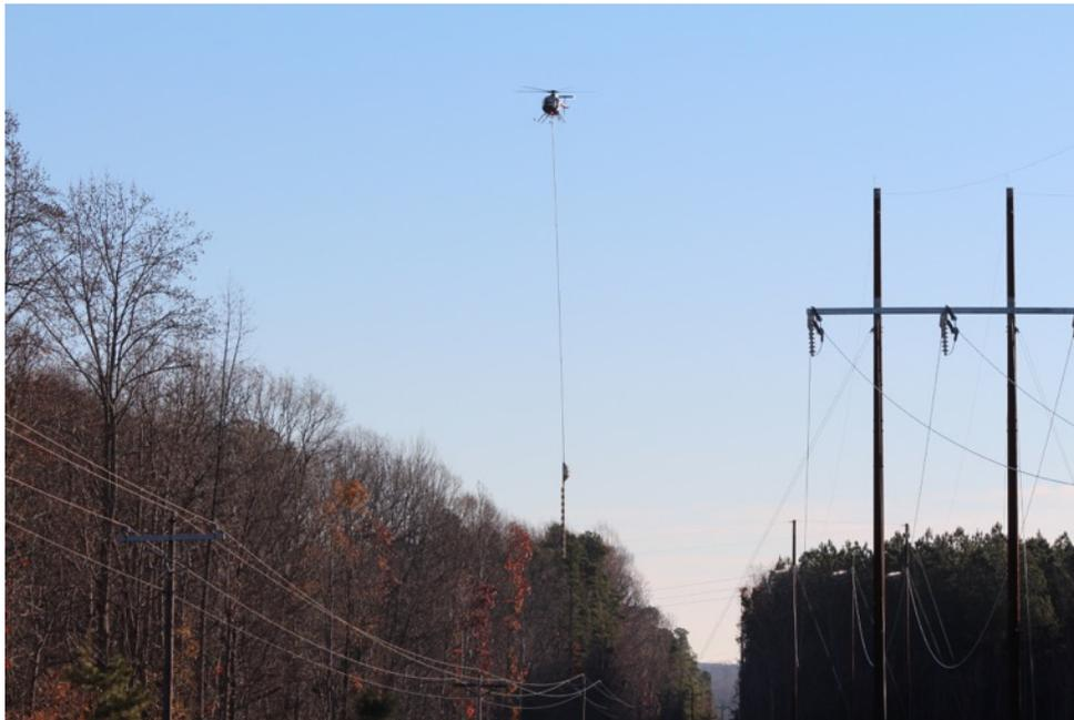
A pilot carefully flies his helicopter above the tall pines, not far from energized electric lines. Dangling under the helicopter from a flexible connecting rod, 10 round, motorized saws controlled by the pilot trim the trees, sending limbs falling to the ground.
