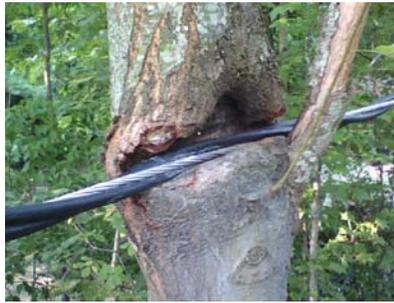
Figure 1 - Tree growing around service wires.
